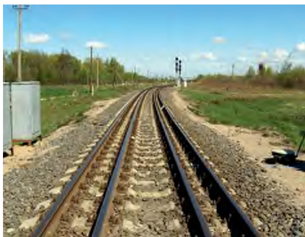
Fig. 1 Dual gauge (1520/1435), Dzerzhinskaya-Novaya station, Kaliningrad. Source: http://parovoz.com
